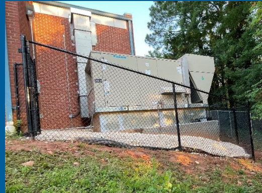
River rock gravel around ground HVAC Units
